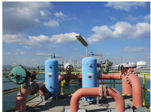
Fire Water Accumulator
